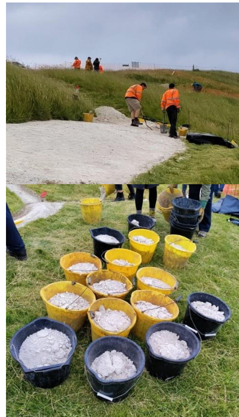
Top, shovelling off some chalk from the belly of the horse to steepen the slope, and, bottom, loading it into buckets to be taken up to the neck and head.
