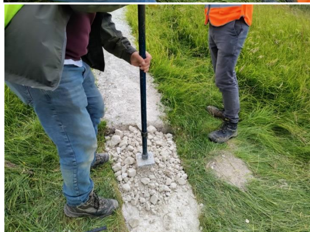
Top, Win Scutt explaining the rationale behind the extension of one of the legs. Below, tamping in chalk to the extension.
