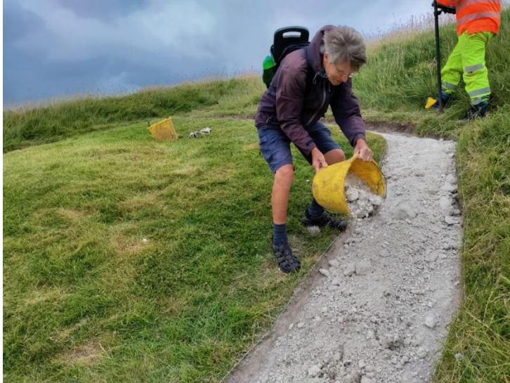
Passing buckets of chalk from the belly of the horse along a chain gang, then depositing it in the newly widened neck.
