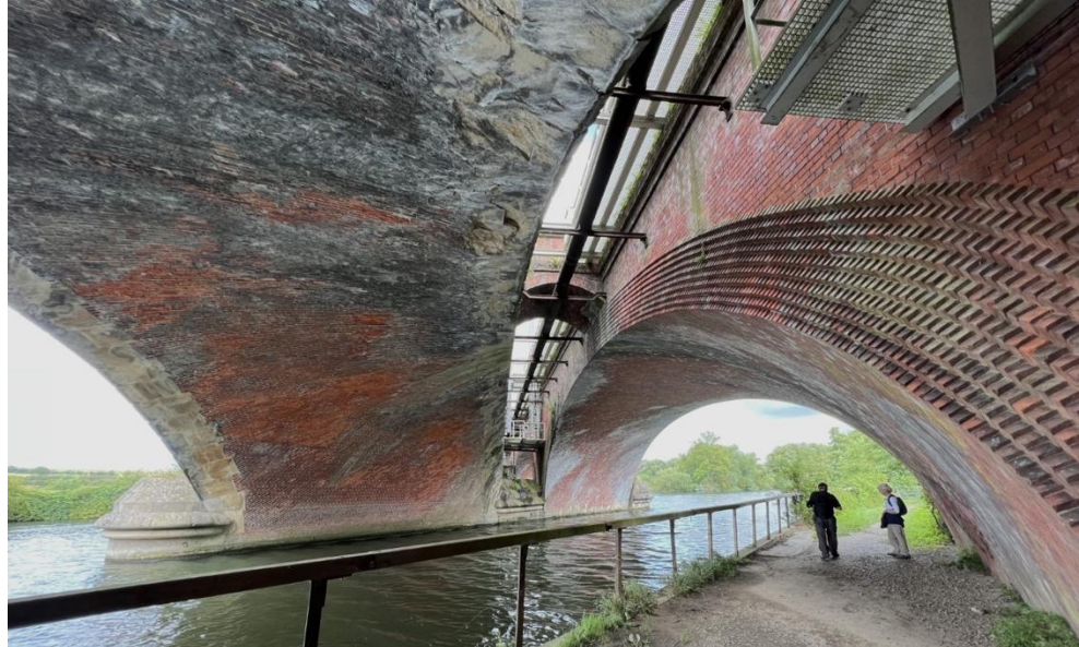
Moultsford Viaduct (Brunel bridge). Photo Sandra Newton
